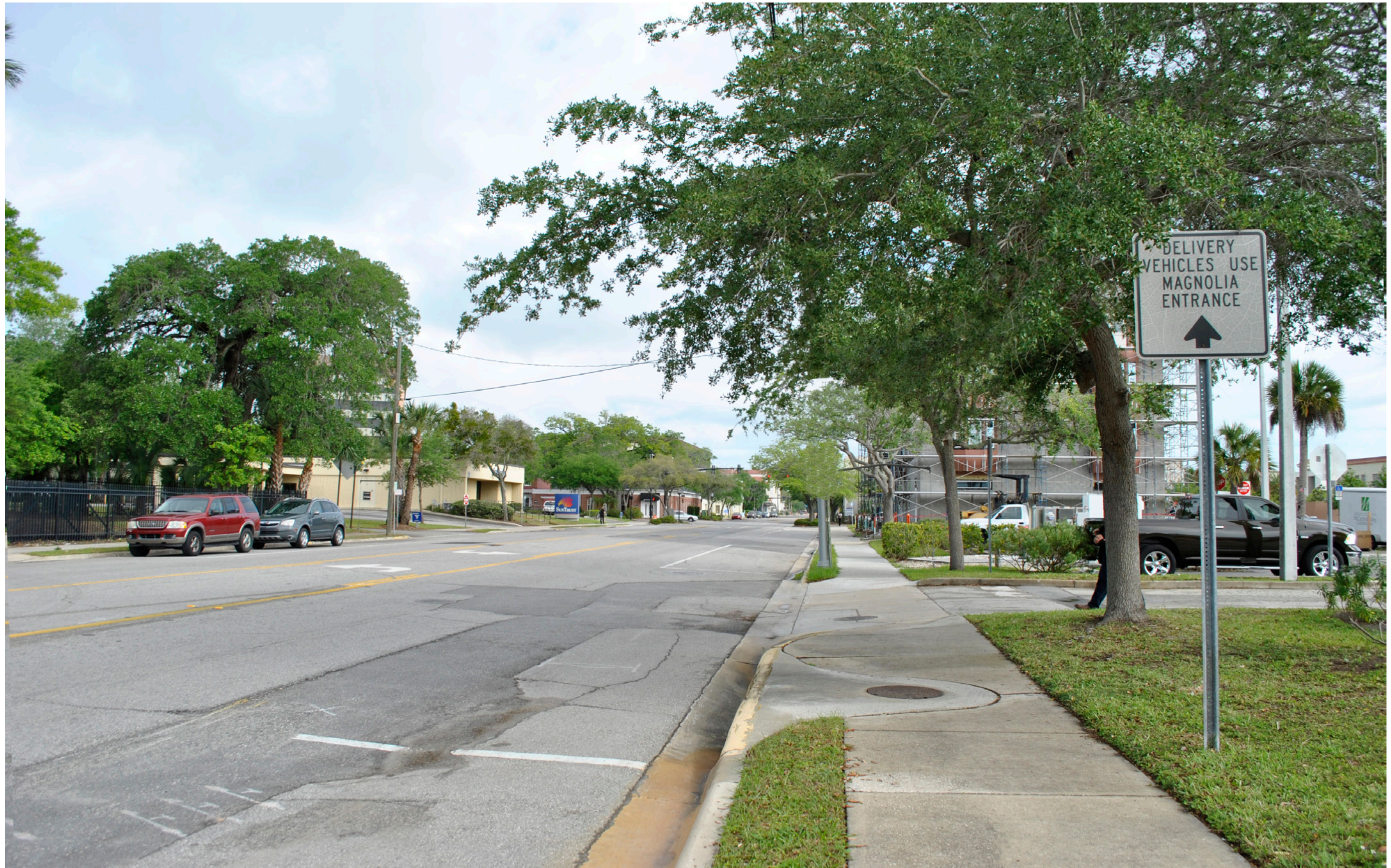
MIXED USE REDEVELOPMENT | BEFORE
